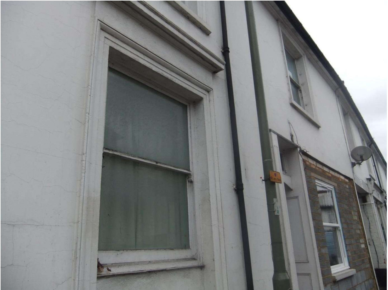
Figure 1 - Photograph of Monitoring Site at the AQMA Addlestone traffic light junction
